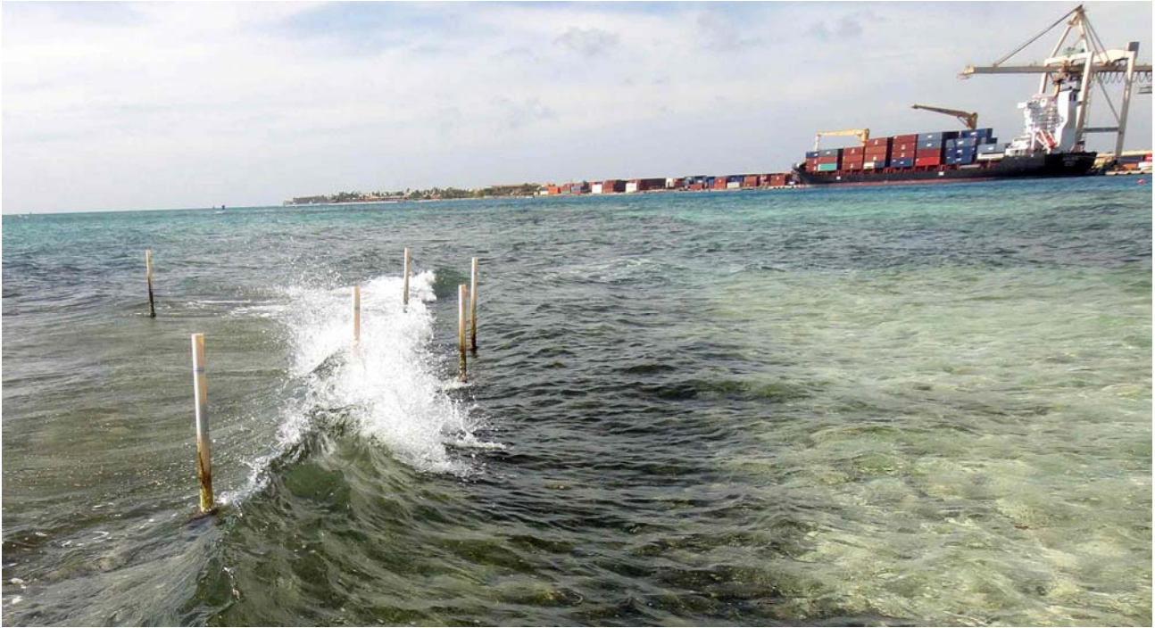
Figure 9 - REM demonstrates resilience to high wave energy on the coral reef
